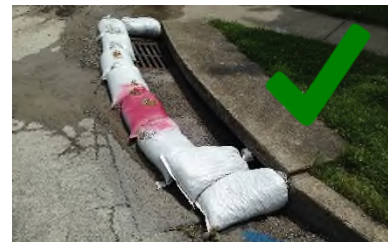
Protect storm drains with rock bags, filter cloth, rock berm, etc.
