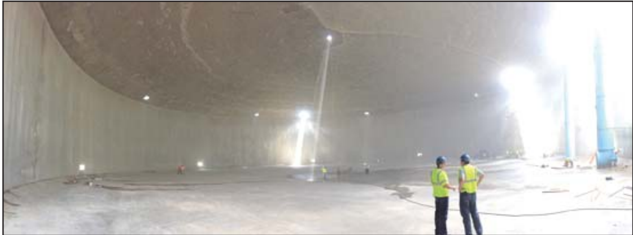
Inside the tank being built at Town Branch Wastewater Treatment Plant
