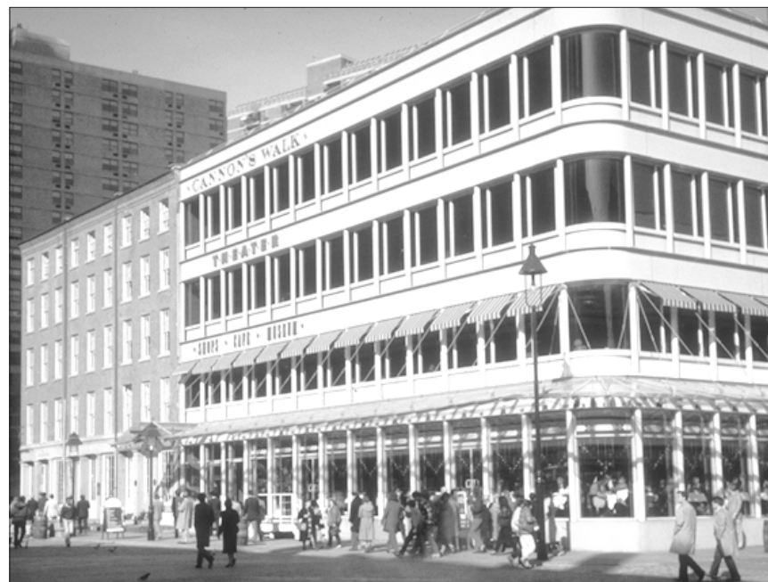
Window sills, moldings and midbelt cornices are among those elements in this new building that align with existing buildings.
