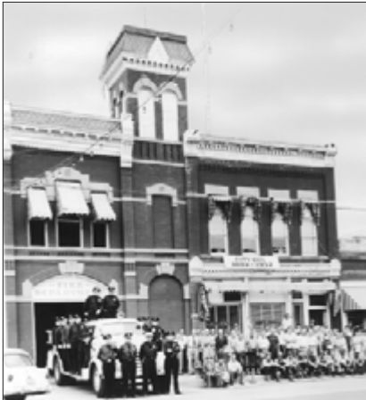
Using historic photographs can help in determining the original character. (Compare with below.)
