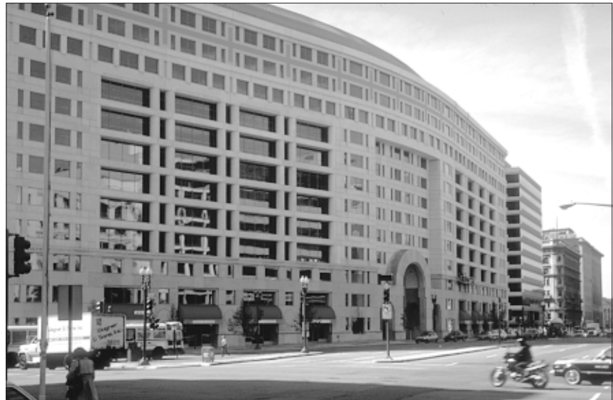
These cast concrete elements convey the scale of traditional masonry facade components, which reinforces the traditional scale of buildings on this street.
