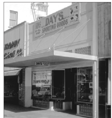
Years later, all original detail had been stripped from the building. (Compare with the photos above and below.)
