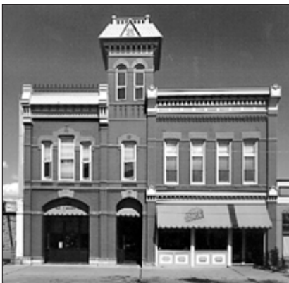
This rehabilitation preserves surviving details and reconstructs missing ones.
