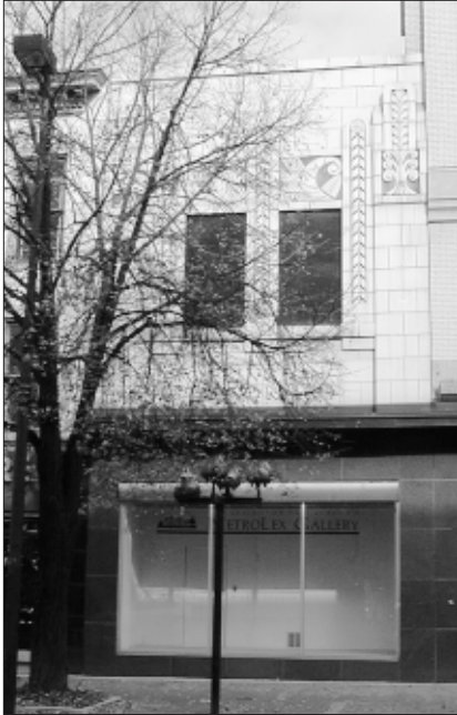
The style is most easily identified by its architectural ornament, which includes stylized floral patterns and repetitive geometric forms incorporating sharp angles and segments of circles.
