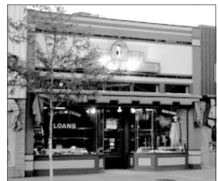
The same building (above) after renovation exhibits the more classical features of commercial storefronts, including a painted cornice, kickplate and recessed entry.
