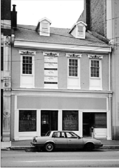
Although window openings have been altered on both floors, this building exhibits the simple forms of Federal buildings. A gable roof, with the ridge line parallel to the street, is a typical feature.
