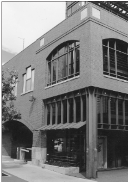
This parking structure incorporates a wrap of retail stores along the street edge. The storefronts are contemporary interpretations of the historic downtown context.
