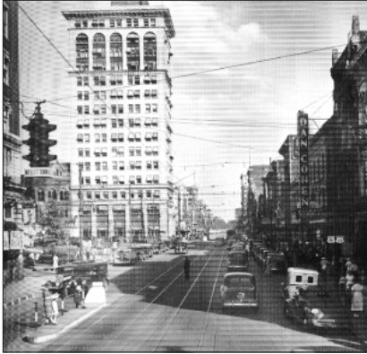
Main Street looking east from Mill. Photograph taken in 1938.
