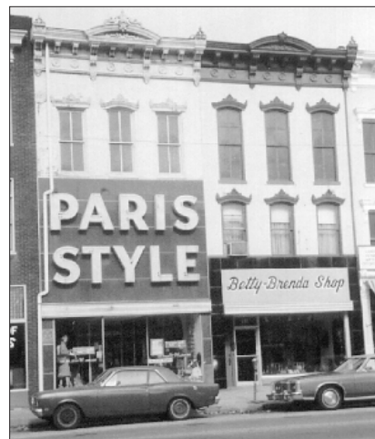
Any sign that visually overpowers the building or obscures significant architectural features, such as this one, is inappropriate.
