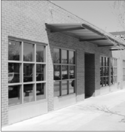
Traditional storefront features—such as a kickplate, display window, transom and recessed entry—are reinterpreted in this new storefront design.
