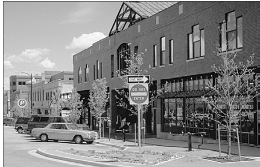
Design a parking structure so that it creates a visually attractive and active pedestrian environment. This parking structure is screened with a two-story “wrap” of retail space.
