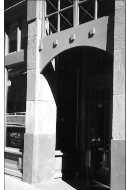
This contemporary interpretation of a storefront includes a recessed entry and transom element.
