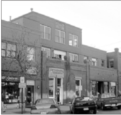
When a rooftop addition is set back from the front, the original scale of the building can be perceived.
