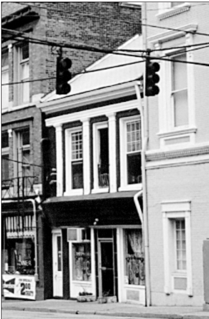
Greek Revival pilasters, or attached columns, adorn the upper level of this structure, which also exhibits the sloping roof form of a Federal period building.
