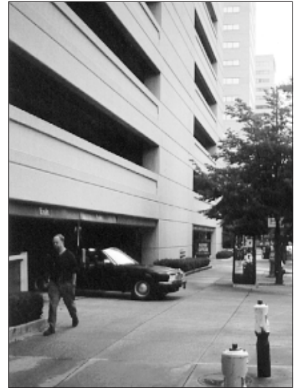
A parking structure should be designed to be compatible with traditional buildings in the surrounding area. This garage fails to do so.
