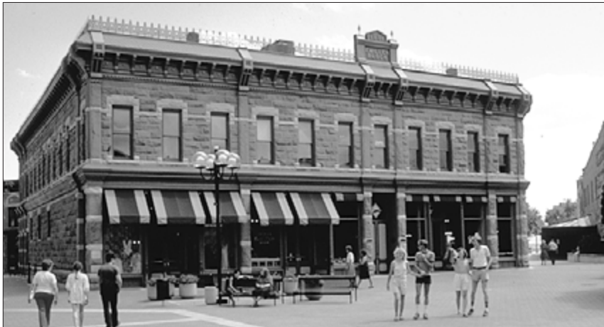
Storefront windows were reopened and upper-story windows were repaired.
