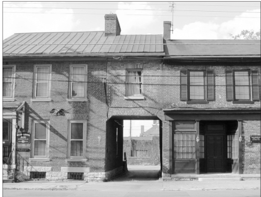
Precedent exists in the area for providing vehicular access that presents less of a conflict with pedestrian movements. The narrow passage in this Federal block of buildings is an example.
