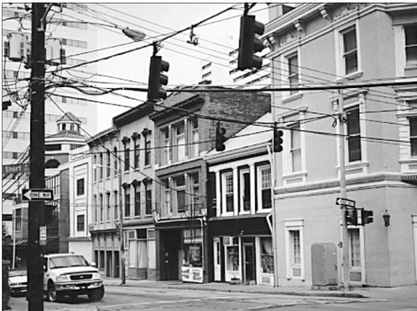
The Courthouse Area conveys a sense of a time and place, which is expressed through its numerous historic and traditional buildings.
