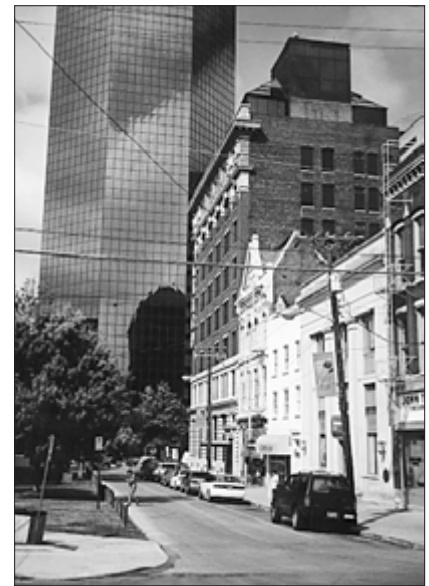
Building heights vary in the area, yet the scale and character of the first floors are quite similar.
