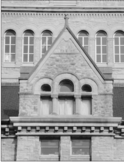
Masonry walls, usually with rough-faced, squared stonework and round-topped arches over windows are typical features of the Richardsonian Romanesque style.
