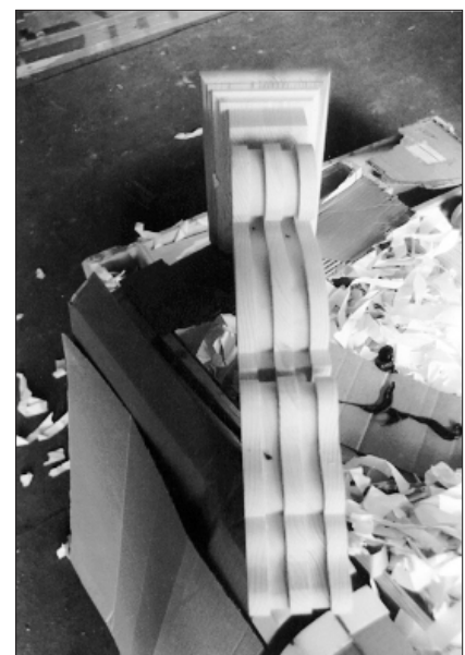
Reconstruct only those portions that are beyond repair.
