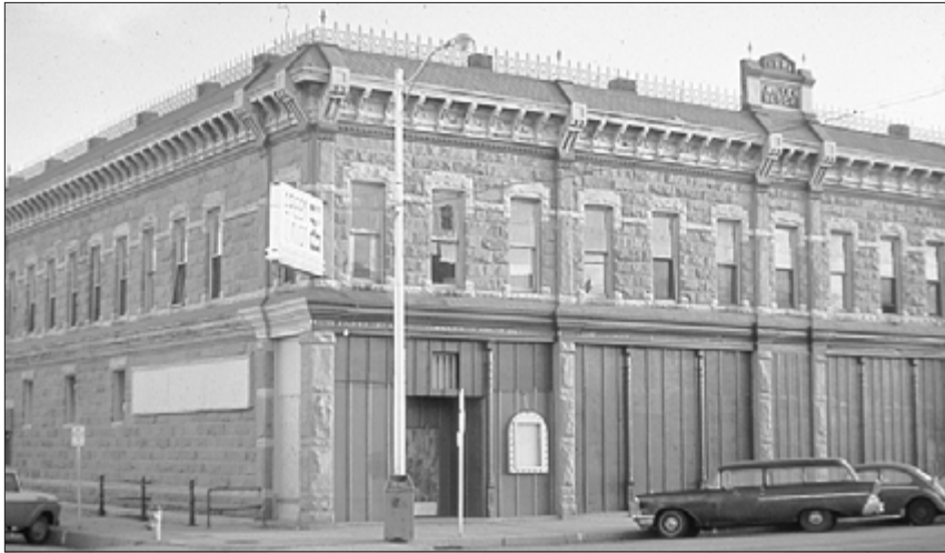
The windows in this structure were boarded and architectural details needed repair. (Compare with the photo below.)
