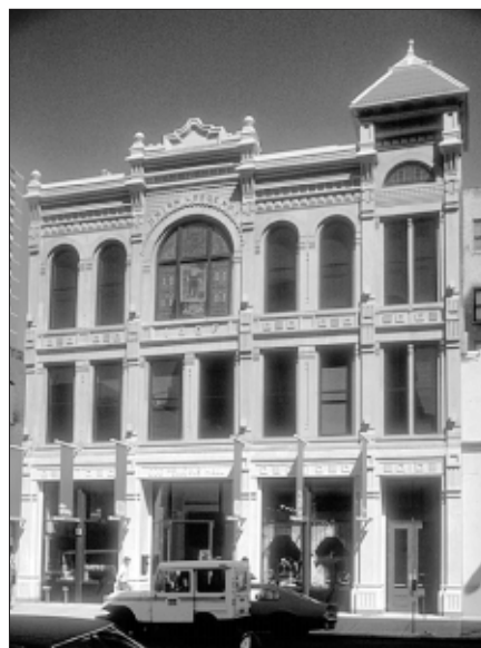
An addition may be set back to preserve the perception of the historic scale of the building. In the image on the left, the original three floors of this building are visible. In the angle view at right, two newer floors are visible. Note how in this building the addition cannot be seen when looking at the building straight-on.
