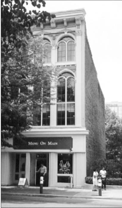
Detail of an Italianate building.
