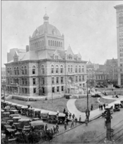
Civic buildings and spaces provide accents in the streetscape.
