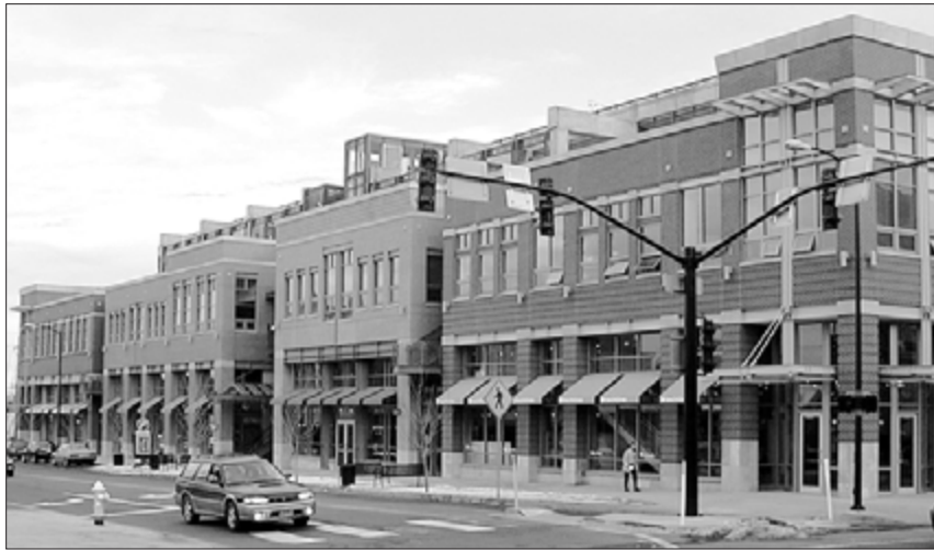
A part of this infill building is a parking structure that is set back from the front and sides of a retail wrap. The openings in the parking section reflect window proportions similar to those seen historically in the area.
