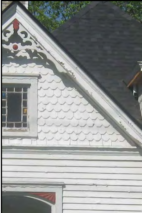
Photo 170: Siding materials such as wood shingles and clapboard should be preserved and maintained (552 East High Street).
