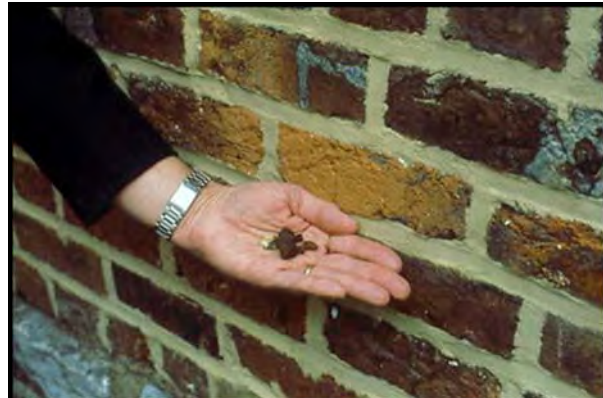
Photos 104 and 105: Hard mortars do not allow brick to expand and contract. ... leading to cracking and spalling.
