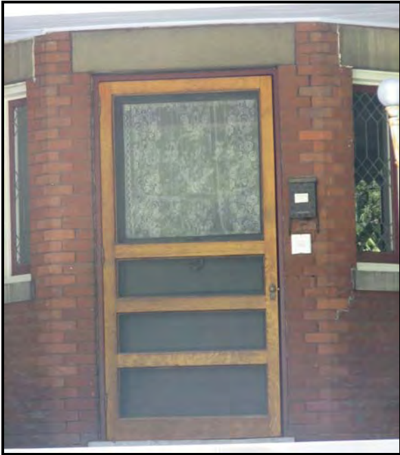
Photo 160: Structural members of this screen door at 444 West Sixth Street are aligned with the wood panels and glazing of the main door.
