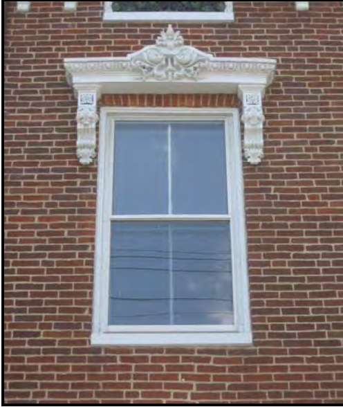
Photo 181: Storm windows should be of full view design or with meeting rails to match the historic window such as at 331 North Broadway.
