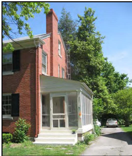
Photos 158 and 159: Screen porch enclosures at 117 Forest Avenue and 323 Arcadia Park maintain the characteristic openness of the porch without obscuring original features such as porch columns.
