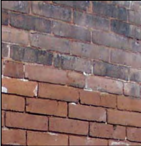
Photos 106 and 107: Brick should be cleaned with detergent or chemical cleaners, not with abrasive, high pressure cleaning methods or sandblasting.
