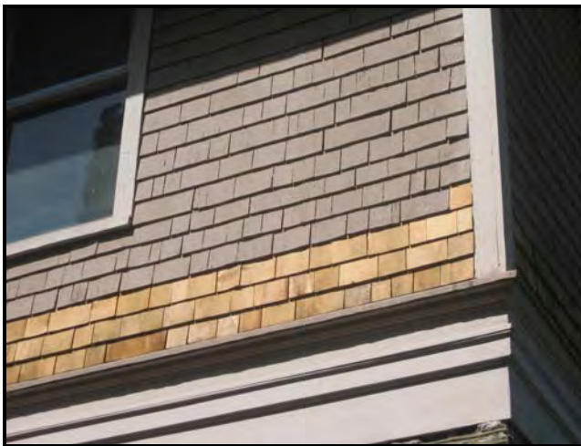
Photo 171: Replacement of siding material such as this wood shingle exterior at 101 Hampton Court, should match the original in size, shape, texture, and other qualities.
