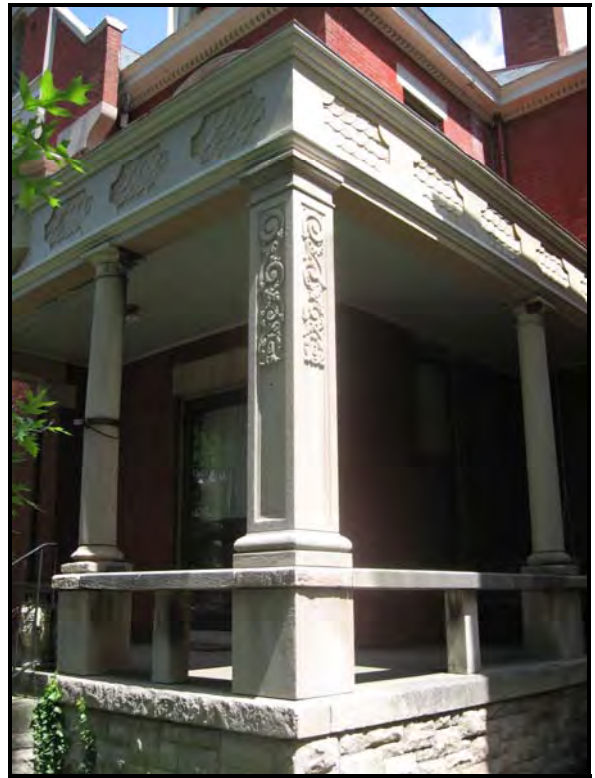
Photo 148: Concrete porch columns at 248 North Broadway.
