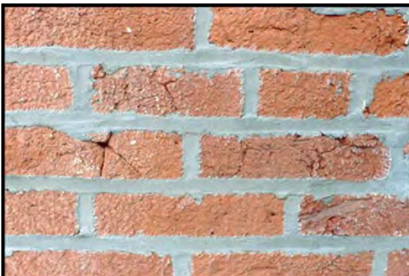
Photos 104 and 105: Hard mortars do not allow brick to expand and contract. ... leading to cracking and spalling.
