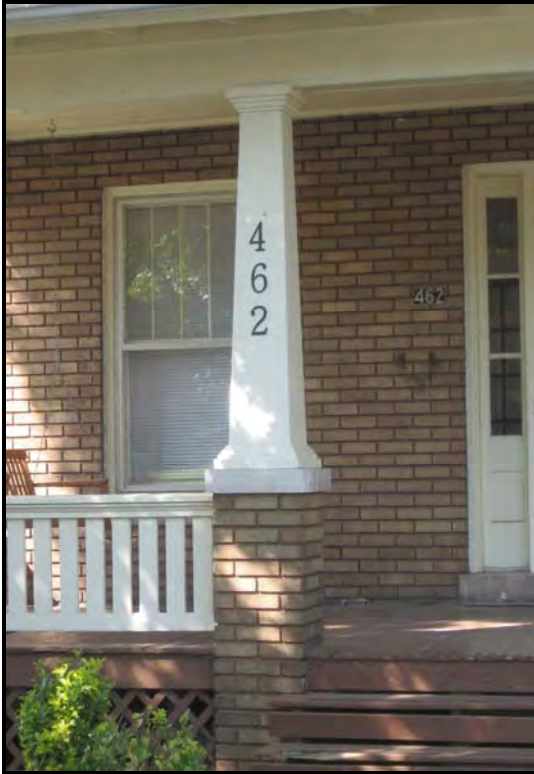
Photo 136: Tapered Craftsman style porch columns at 462 East Maxwell Street.
