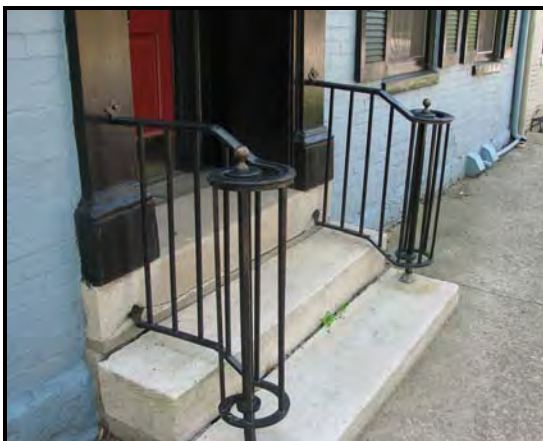
Photos 109 and 110: Cast iron elements should be preserved and maintained (344 South Upper Street and 176 North Broadway).
