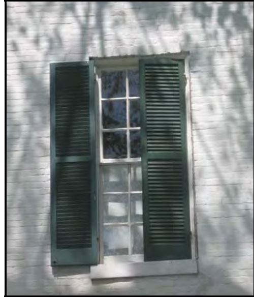
Photo 166: Proper shutter fit 471 West Second Street.
