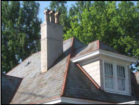
Photos 149, 150: Original slate roofs should be preserved, maintained and repaired (265 South Ashland Avenue, 332 Aylesford Place).
