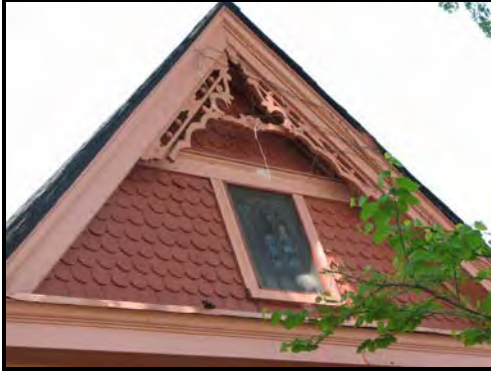
Photo 95: Preserve and maintain elements such as eave bargeboard (315 South Mill Street).
