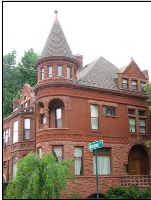
416 West Third Street demonstrates the use of textured masonry of various shades to create decorative wall patterns.
