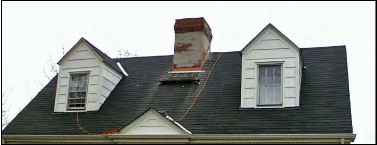
Photo 116: Proper repair and flashing of chimney on Barberry Lane.
