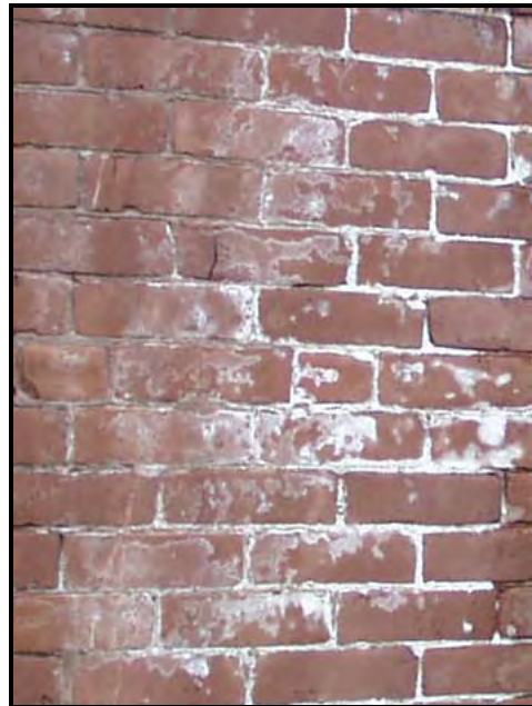
Photos 106 and 107: Brick should be cleaned with detergent or chemical cleaners, not with abrasive, high pressure cleaning methods or sandblasting.
