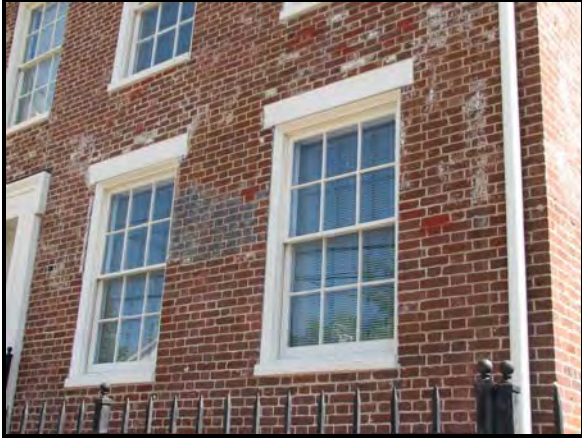
Photo 184: Appropriate window replacement of six-over-six wood sash windows. (609 West Main Street)
