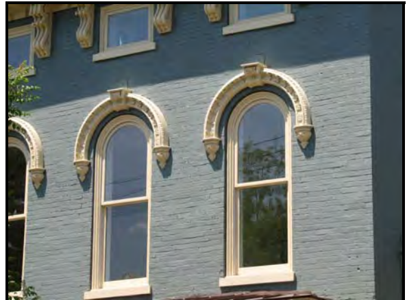
Photo 100: 355 South Upper Street Original window trim and moldings should not be removed or concealed.
