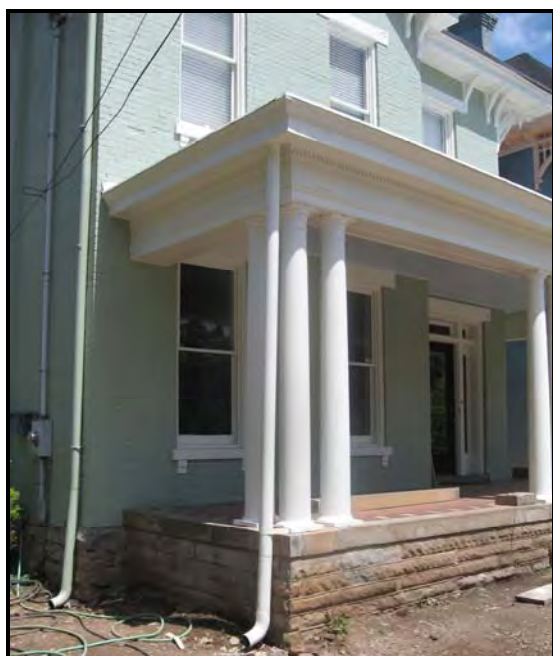
Photo 132: Proper downspout placement at 417 West Third Street.
