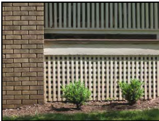
Photos 126 and 127: Lattice panels are appropriate and recommended for infill between brick pier foundations and should be added between piers not in front or behind them (332 Hampton Court, 444 Fayette Park).
