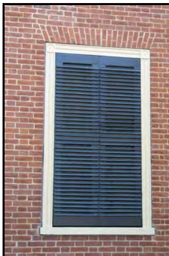
Photos 164 and 165: Examples of both opened and closed shutters at 231 North Mill Street demonstrate the proper fit of shutters to windows. Note the correct attachment to the window frame as well.
