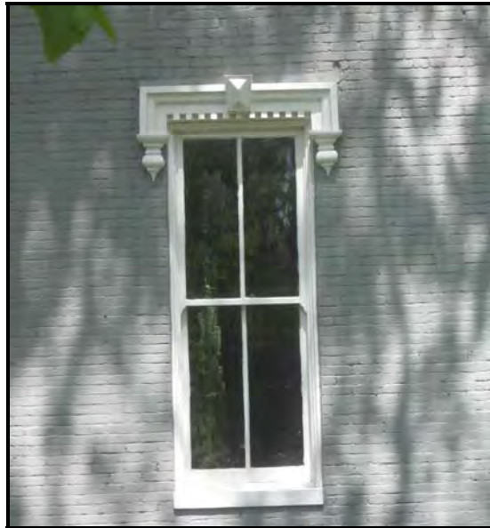
Photo 185: Original two-over-two sash window at 445 West Third Street.
