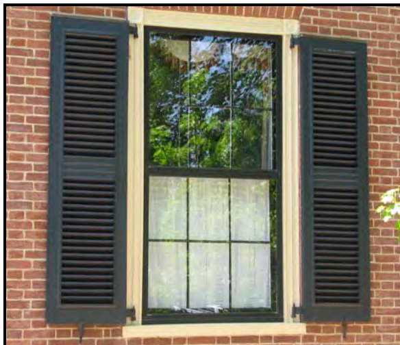
Photos 164 and 165: Examples of both opened and closed shutters at 231 North Mill Street demonstrate the proper fit of shutters to windows. Note the correct attachment to the window frame as well.
