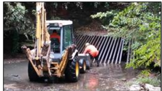
"Critical" culvert locations routinely inspected and cleaned by LFUCG to reduce flooding.
