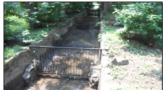
A backhoe is used to remove debris at the Parkside Cave stormwater grate (top). However when some sites get clogged, such as the trash screens at Lexington Cemetery (middle), the Storm Crew must remove the debris using hand tools to allow the water to drain (bottom).
