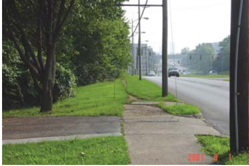
Sidewalk ends along an arterial road
