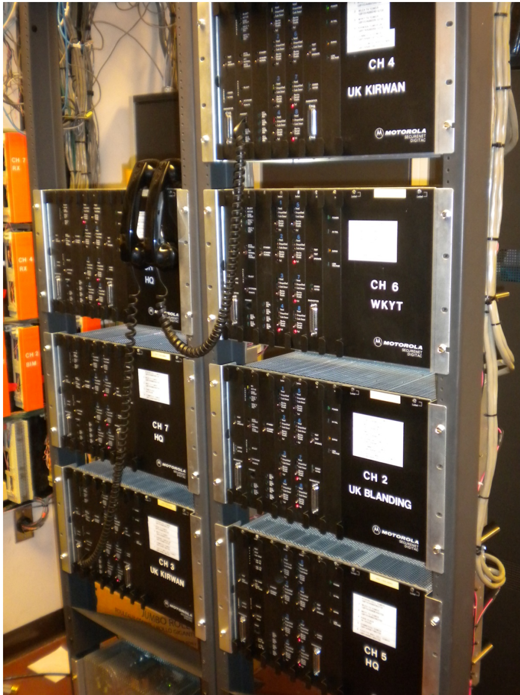
Figure 2 – Motorola Securenet – comparator for satellite receiver conventional system used by Division of Police.
