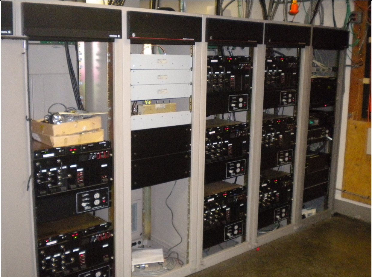
Figure 1 – EDACS repeaters, combiners and Site Controller at the Patterson Office site at UK
