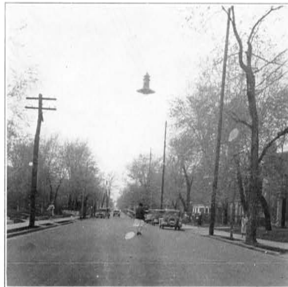
SUSPENDED LIGHTING UNIT (600 candle power light)
