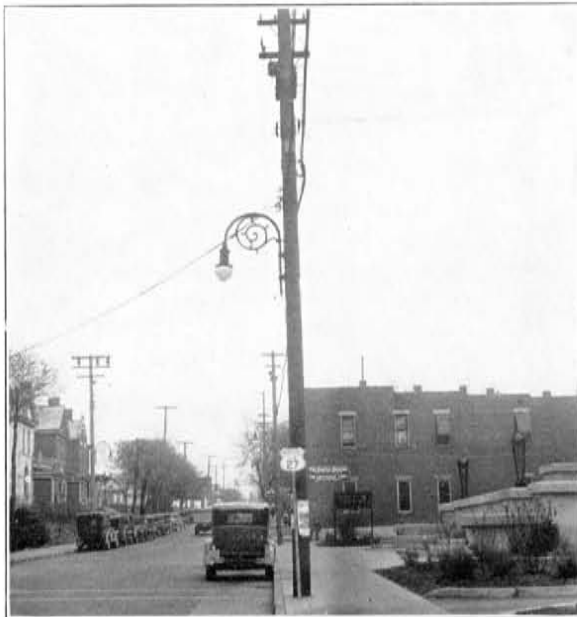
ORNAMENTAL BRACKET ATTACHED TO WOODEN POLE (1000 candle power light)
