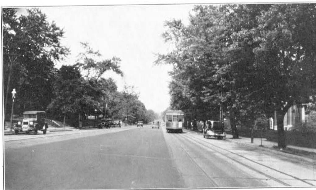
STREET CAR TRACKS IN THE OUTER TRAFFIC LANES 80 foot street, 56 foot roadway
