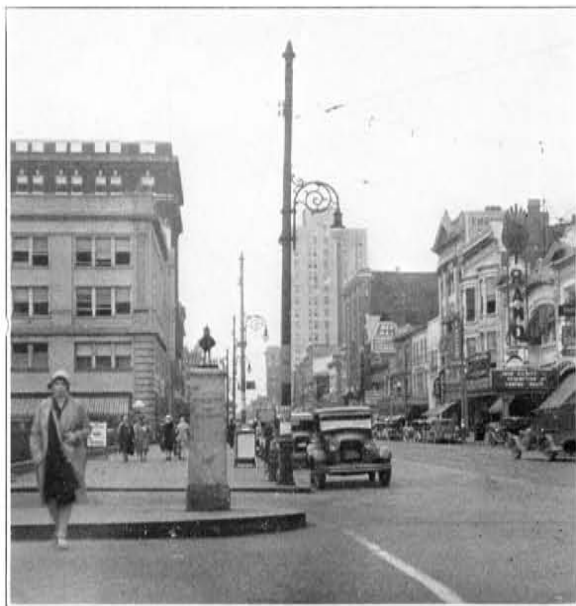
ATTRACTIVE LIGHTING UNITS (Note attaching of all wires to lighting poles)
