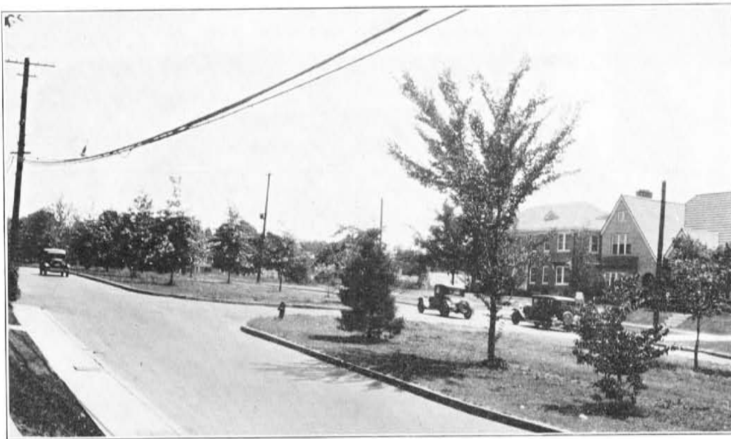
TWIN ROADWAYS AND CENTER PLANTING ON RICHMOND PIKE 120 foot street — 20 foot roadways
