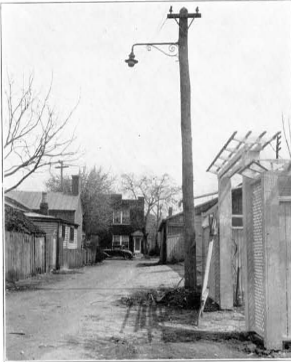
ALLEY LIGHT IN RESIDENTIAL SECTION (250 candle power light)
